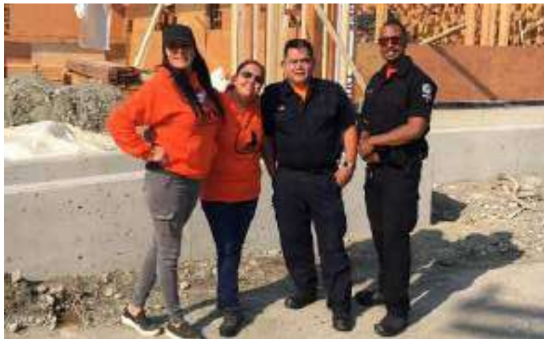
New office building site in Mount Currie on Orange Shirt Day, September 30, 2020.
